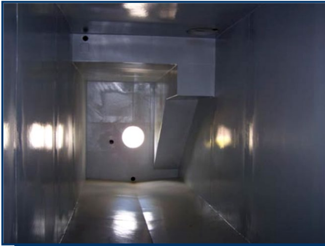
Interior view of smooth walls and "V" bottom
